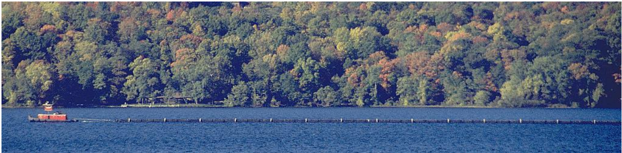
Autumn tow of 63" (1.6m) pipeline for an air-conditioning intake at Cornell University
