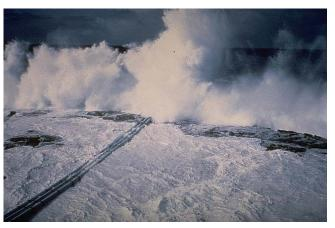
bottom. The pipeline was installed in 1981 off Keahole Point, Hawaii. In spite of its "temporary" design life of 2 years, it has survived many major storms including a hurricane and was operational for over twelve years.
