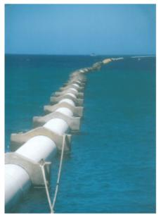
40" Intake Pipeline Design and In a project with R.M. Installation: Towill Corporation, funded by the State of Hawaii and the U.S. Department of Energy, Makai was tasked with the design of a 40" polyethylene cold water pipe to be used jointly by the Natural Energy Laboratory and the Hawaii Ocean Science and Technology (HOST) Park sites on the Big Island. It is the largest deep-water intake pipeline in the world. This pipe is a larger and more rugged version of the
