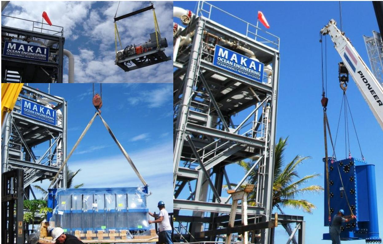
*Makai has installed two new heat exchangers and a turbine-generator, which will complete the OTEC power cycle.*
